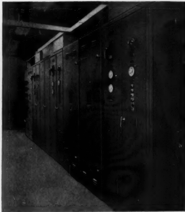
FULLY AUTOMATIC PANEL combines power and control circuits for the d-c drive motors in this compact row of cubicles. For any future plant expansion, matching cubicles can easily be added.
